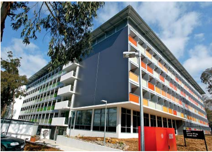
View of the completed Laurus Wing of Ursula Hall at the ANU.
